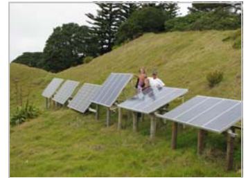
IMG6: ADJUSTING THE SOLAR ARRAY ANGLE
